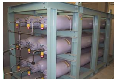
Hydrogen storage tanks 110MPa, 72L x 9
